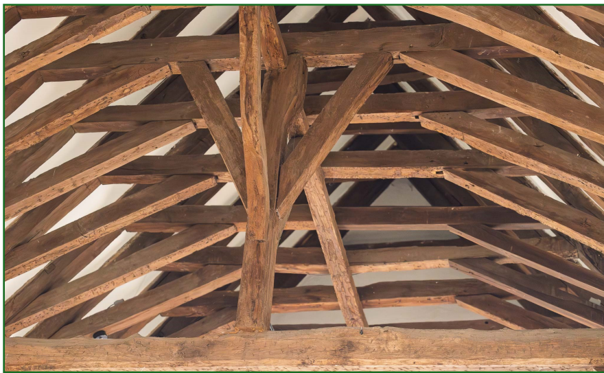
Chancel roof—crown post construction (dm)
