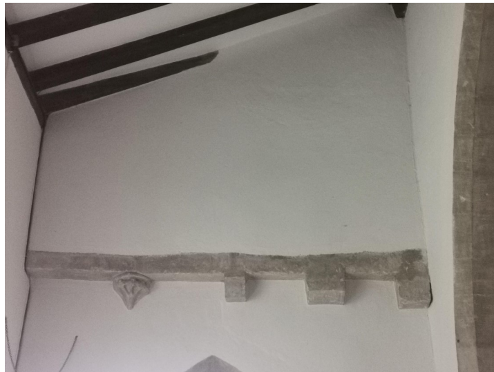
North transept interior from the aisle (ar-m)
