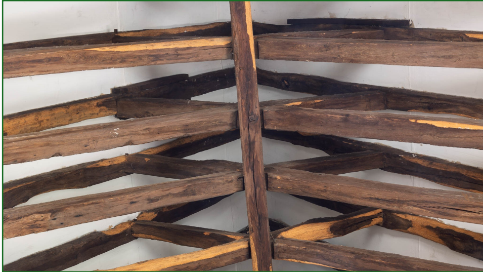
Above: scissor brace roof; below lancet windows (dm)
