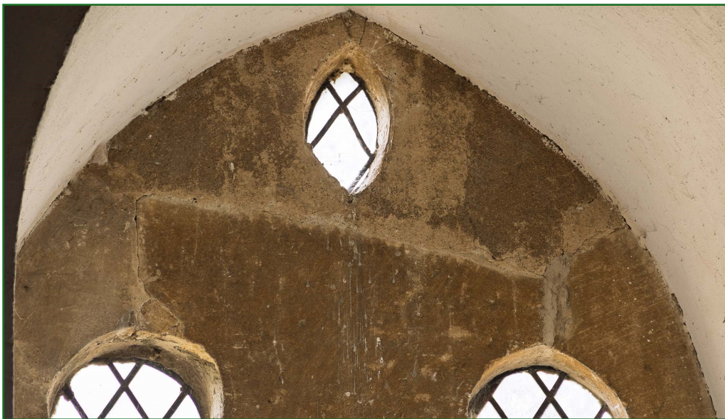
Plate tracing in the West window (dm)
