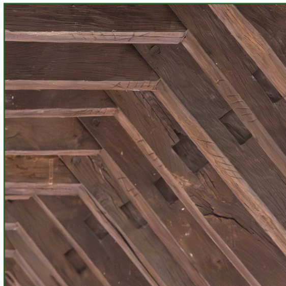
Roof beams The trusses in the roof apex, show trusses number X to XIII, noting the detail of the scratched numbering (dm)
